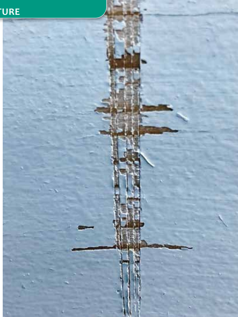
Test de quadrillage
